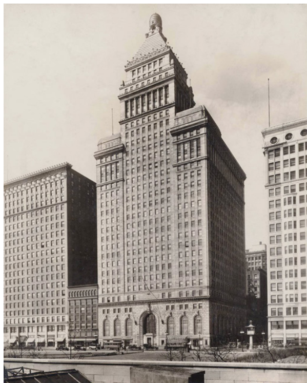
Figure 2. The Straus Building, located at 310 S. Michigan Avenue, Chicago, IL (corner of Jackson and Michigan). Photograph from the Art Institute of Chicago's Ryerson & Burnham Historical Archival Image Collection.
