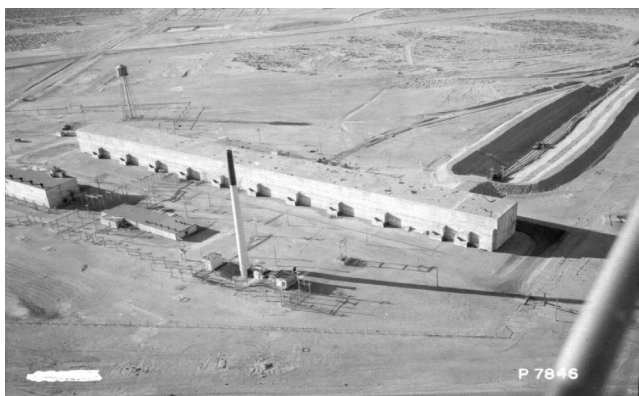
Figure 6. T Plant, Hanford, based on bismuth phosphate coprecipitation (long building at center) and lanthanum fluoride (building at the left), operated 1944-1956. Photo taken 22 December 1944, during initial start-up operations. Taken from archival original of Ref. 15.
