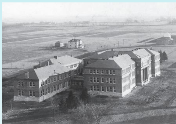
Davenport Hall aerial view, 1900. Note the Observatory in the upper right.
